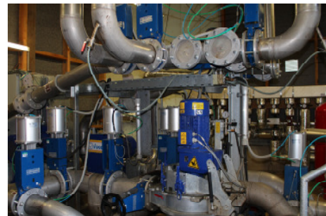
Figure 7: Pumps and pipes between the fermenters
