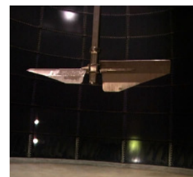
Figure 2: Example for central/axial stirring (for technical reasons not from the plant Miller). Photo: DLZ
