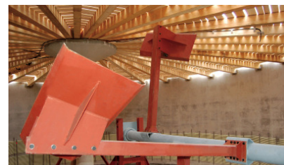
Figure 10: Stirring equipment “Paddelgigant” (company photo, not on Krumbeker Hof). Photo: Agrikomp
