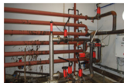
Figure 3: External heat exchangers for the substrate.
