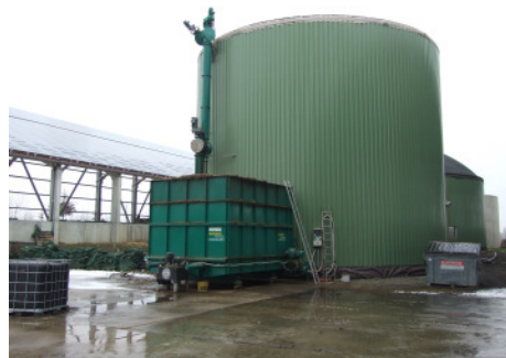
Figure 1: Feeder and first fermenter. To the left is the covered silage storage.
