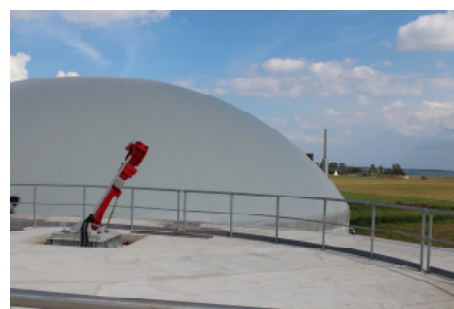
Figure 6: Fermenter with concrete roof and digestate storage with foil roof
